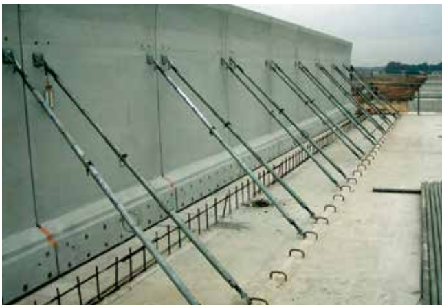
橋梁の高欄部型枠
