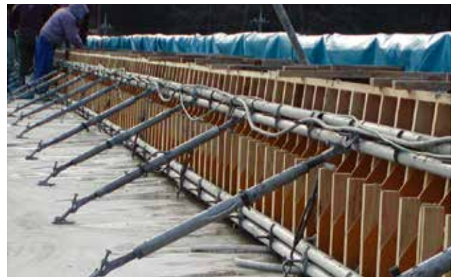
橋梁の高欄部型枠
