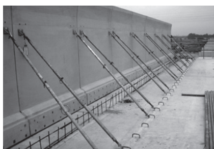
橋梁の高欄部型枠
