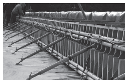
橋梁の高欄部型枠
