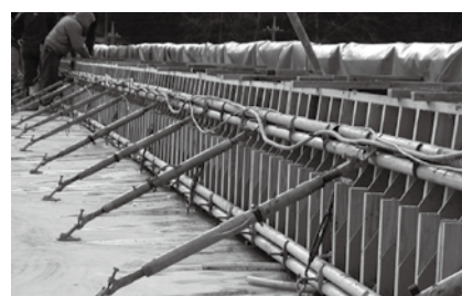
橋梁の高欄部型枠
