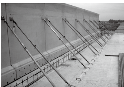
橋梁の高欄部型枠
