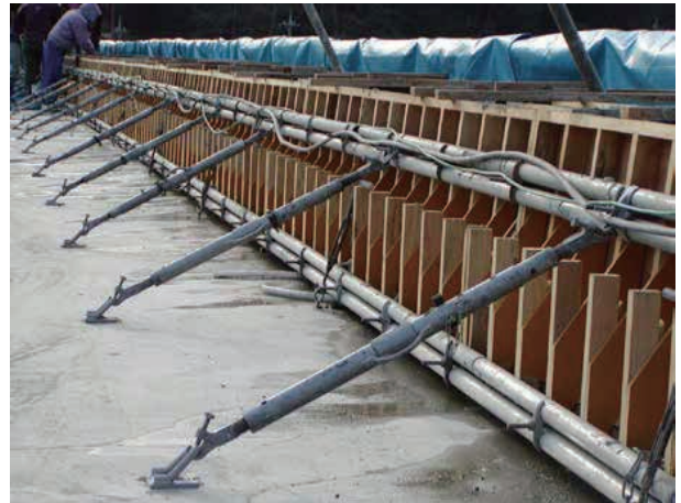
橋梁の高欄部型枠
